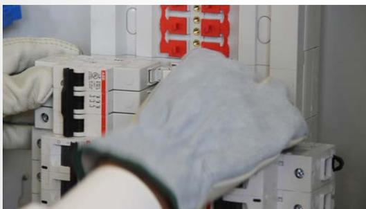
The Breaker Snaps Into The DIN Rail
