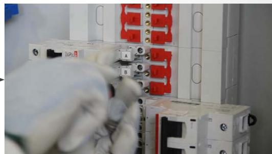
The Breaker Is Secured With An Isolated, Non Conducting Screw
