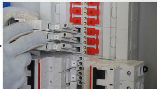
The Breaker Is Inserted Into The Opening
